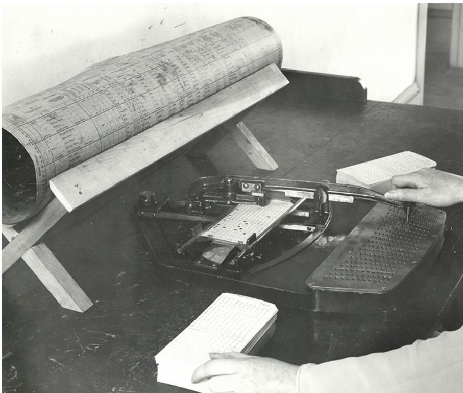
A pantograph used in the 1931 Census to punch cards
